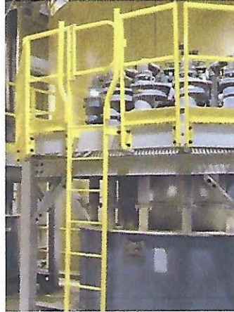
Raised platform with protected guardrail.
